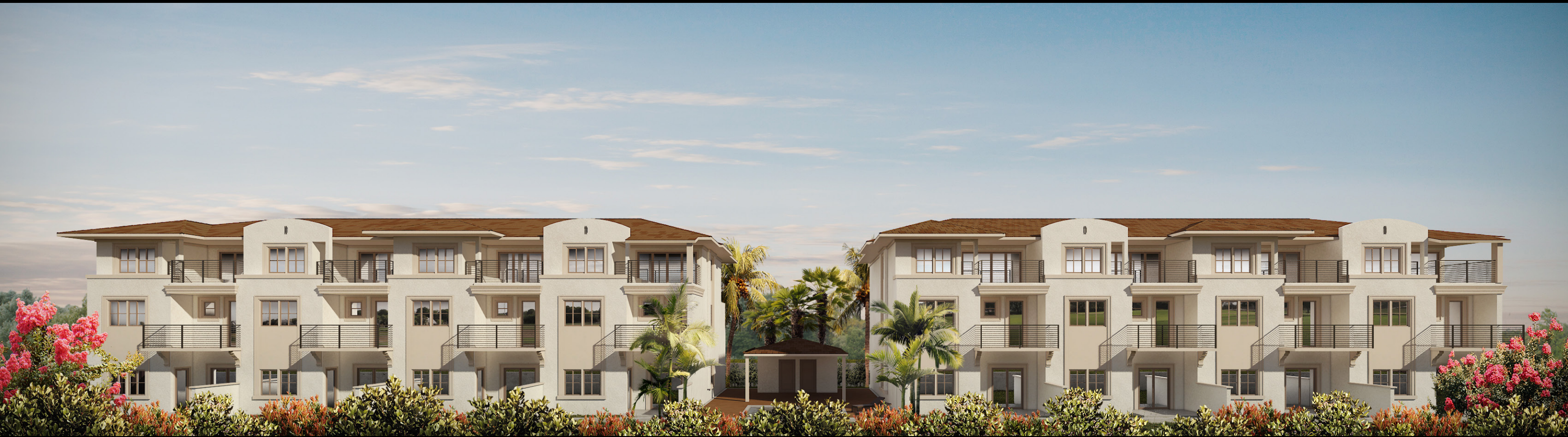
Rear view of Seaview Ridge
